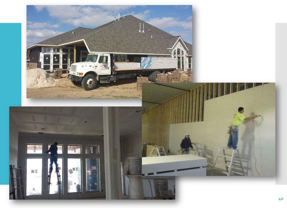
Sheetrock is a milestone because all of the mechanicals in the walls must be finished and insulation must pass a third party inspection.
